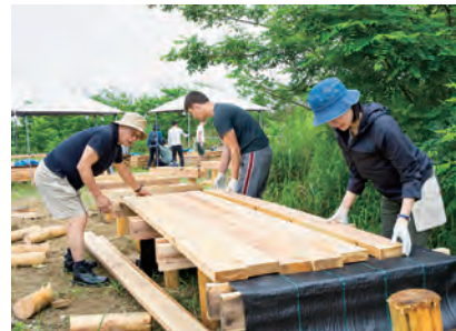
4 床面となる木材を並べます Planks of wood were lined up to create the walking surface.
