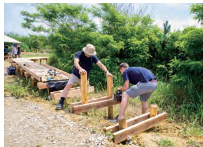
6 木道の始まり部分は道と地続きになるよう設置 The first section of the path was installed so as to join the ground smoothly.
